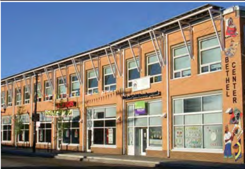
Bethel Center houses a bank, Head Start classes, day-care and employment services, a dry cleaners, and a sandwich shop in a convenient location next to the rail station.
